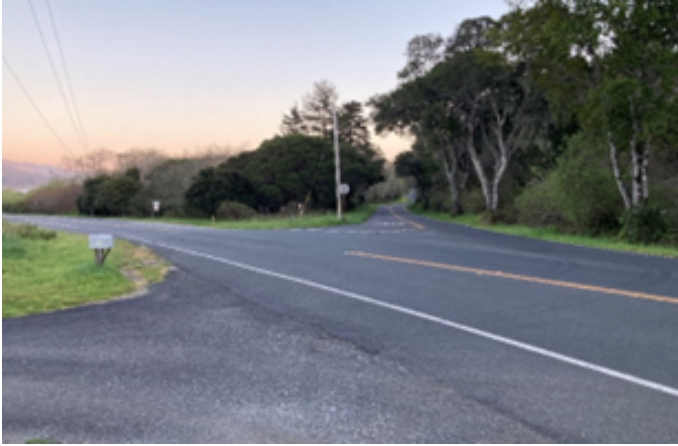
The Intersection of SR-1 and Olema Bolinas Road, looking south from SR-1.
