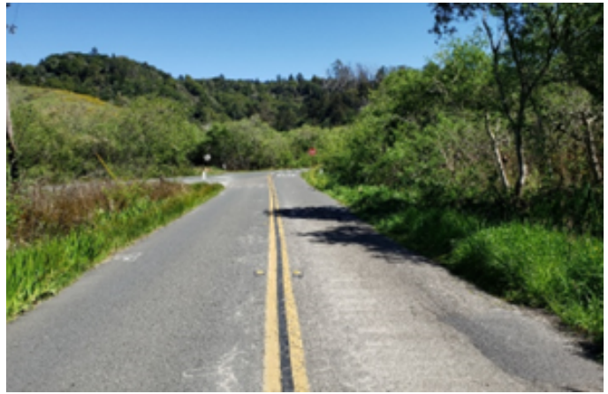
Fairfax Bolinas Road within the Project site, looking toward SR-1.
